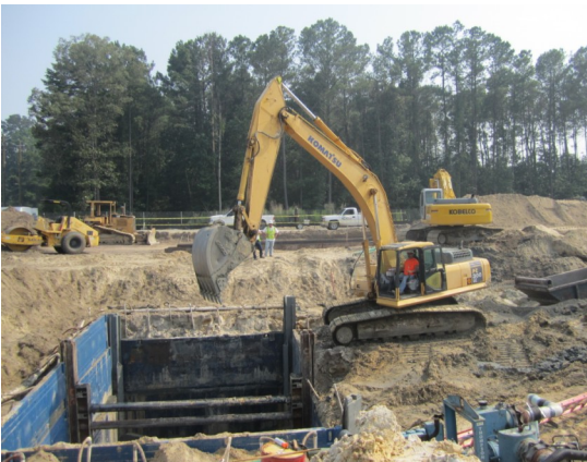
Left: Excavators have been working for weeks digging a massive hole to house an Emergency Sewer System.
